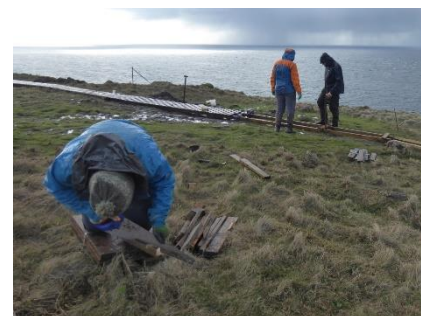
Boardwalk construction underway
