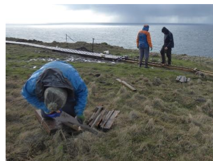
Boardwalk construction underway
