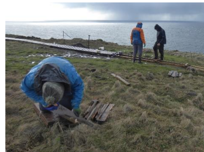
Boardwalk construction underway
