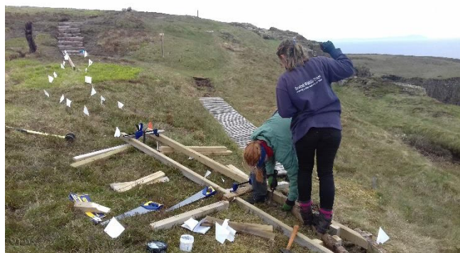
A new section of boardwalk under construction.
